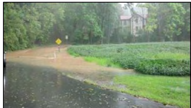
Figure 5.2.1.1-1: Flash Flooding, Hellam Township 2012
