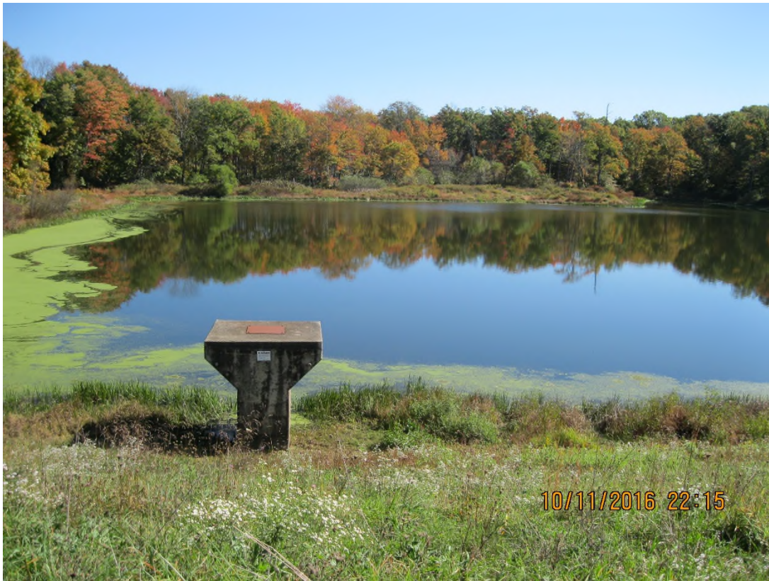
Figure 4.3.2-1. Koenigs Creek Dam
