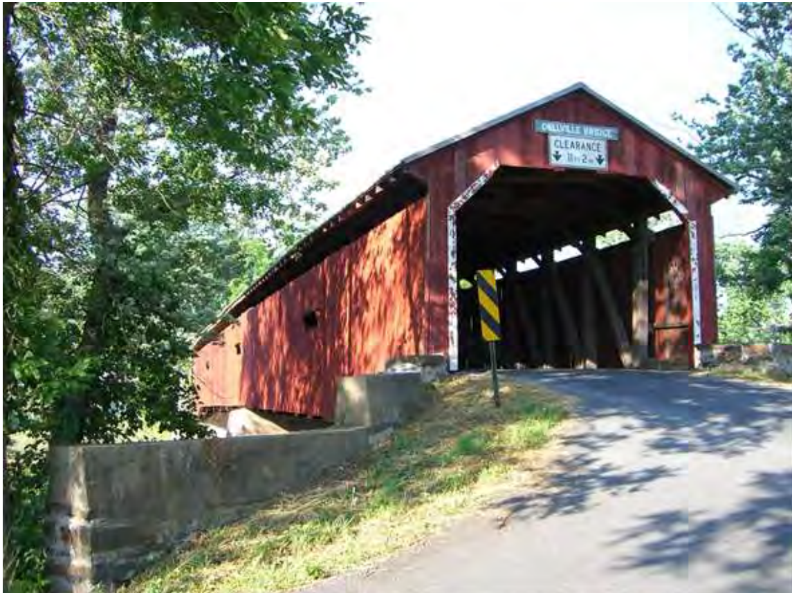
Dellville Bridge before arson fire
