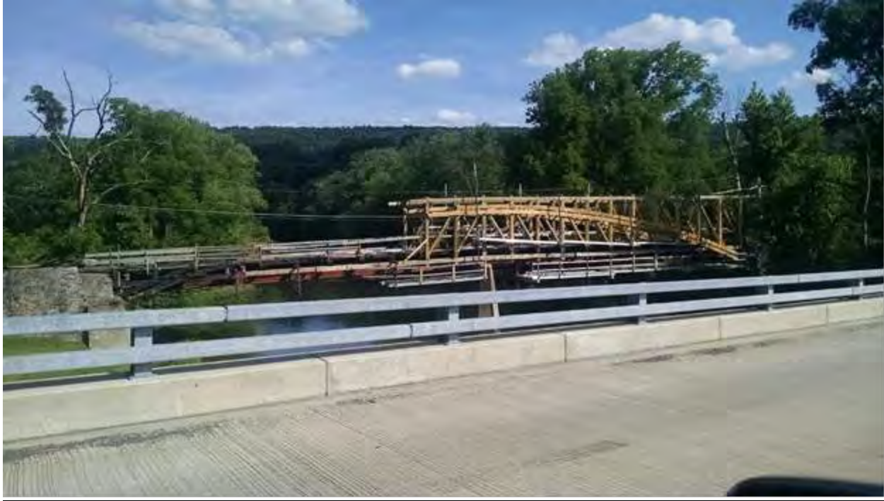
Reconstruction work commencing on the Dellville Bridge following the arson fire
