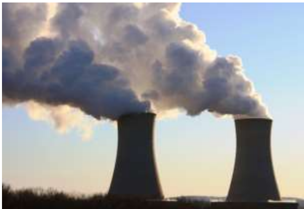
Limerick Nuclear Power Station
