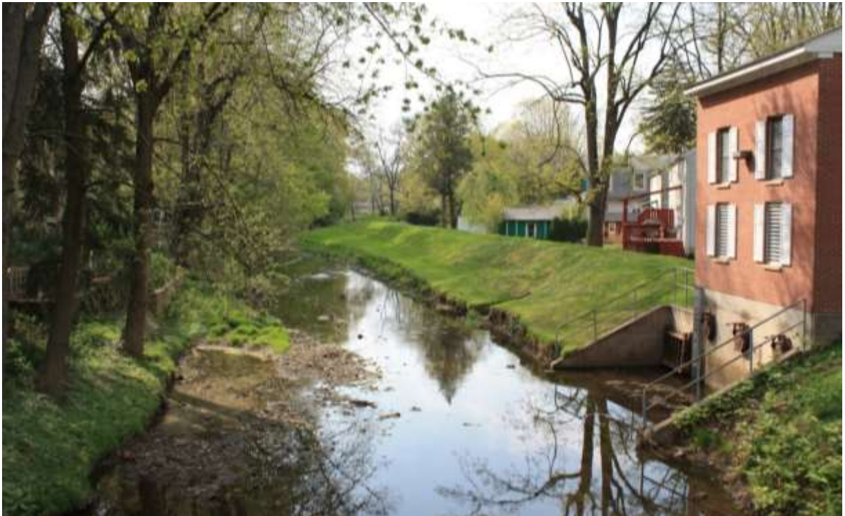
Stormwater pump station on the Tookany Creek
