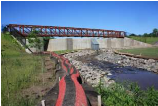
Flood control structure in Upper Dublin Township
