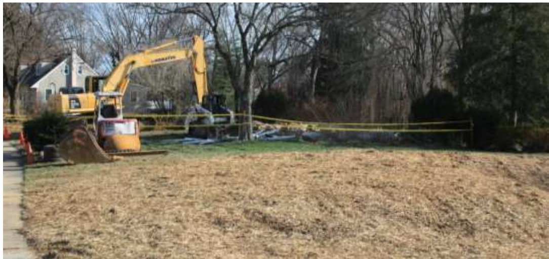
Site grading after removal of a repetitive loss structure.
