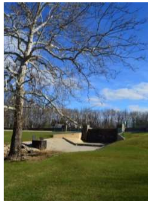
Loch Alsh Dam spillway
