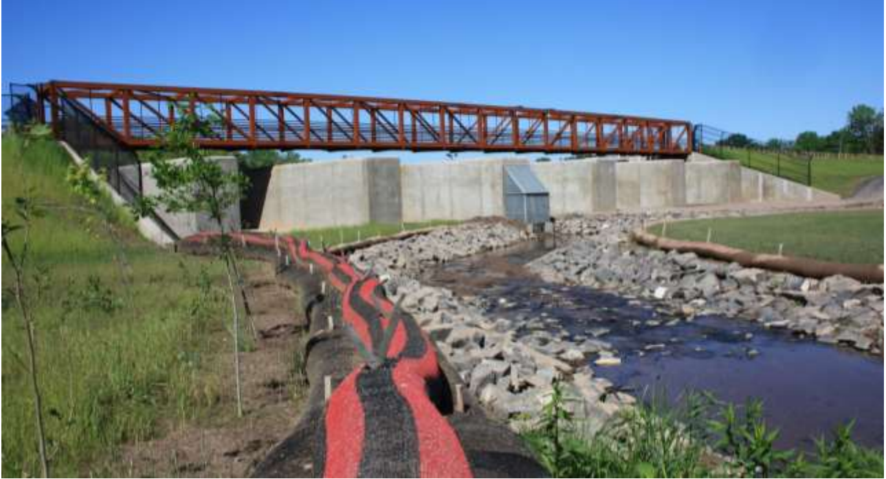
Flood control structure in Fort Washington Business Park
