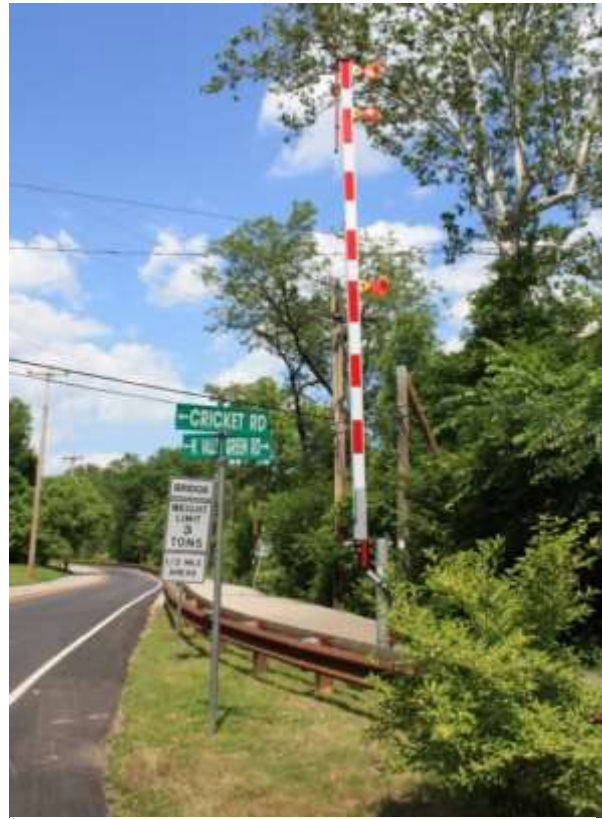
Flood warning gates in Whitemarsh Township
