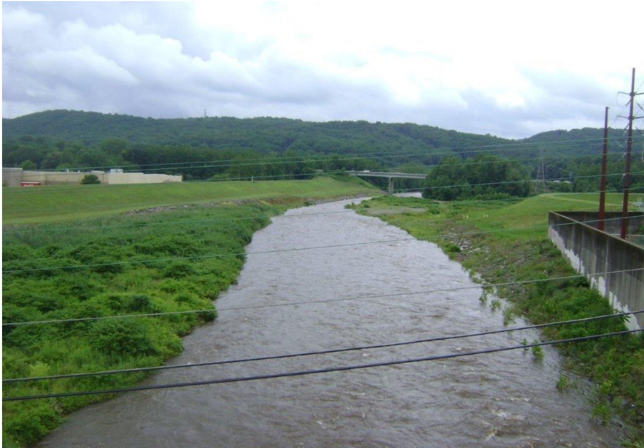
Figure 44 - Stormwater Flowing Through a Monroe County Levee
