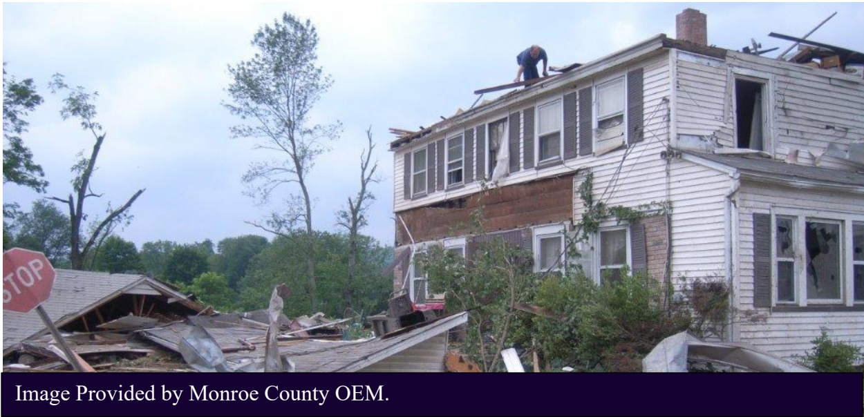
Figure 34 - Property Damage is Assessed Following a Tornado
