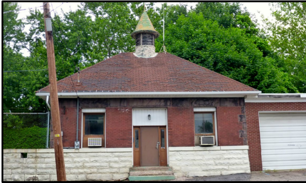
The former Office of the Spring Book Water Supply Company. Source: FEMA EHP.
