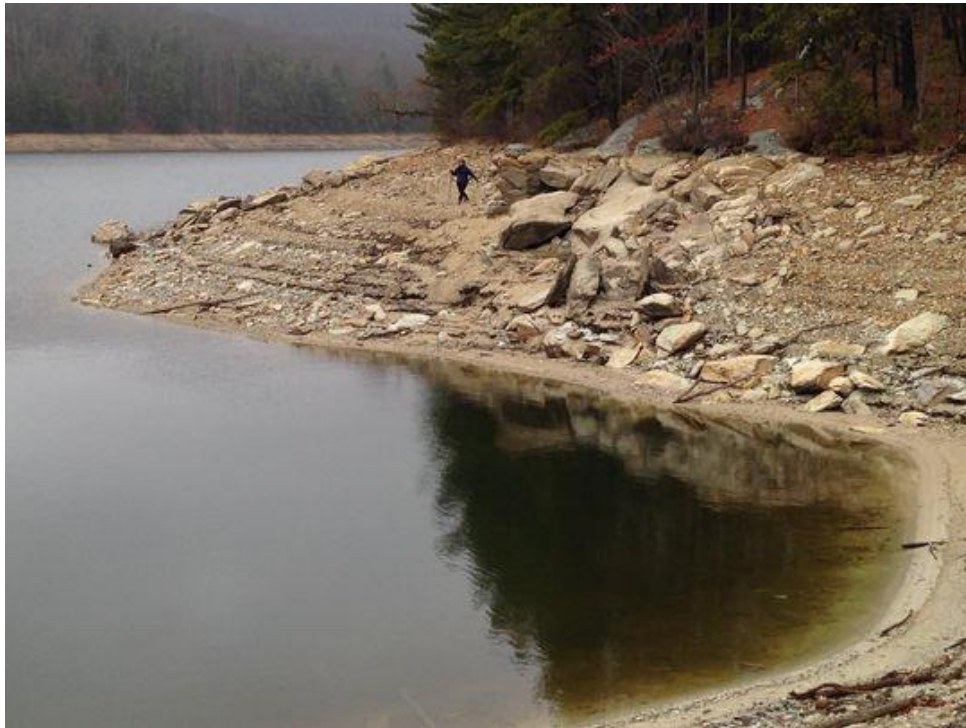
Figure 4.3.3.3.1: Long Pine Run Dam Drought Impact (Dec 2016)
