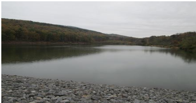
Figure 4.3.2.5.8: Whitetail Land Co. – A Dam Entrapment Area
