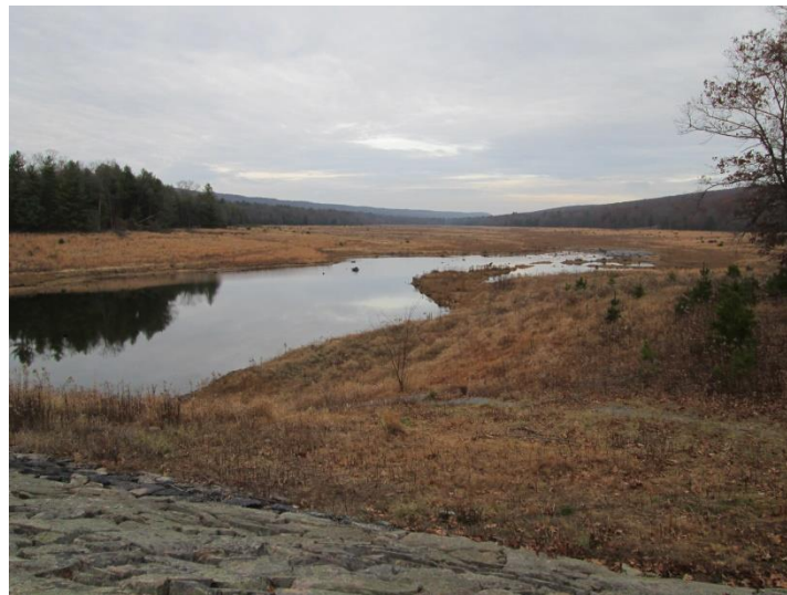
Figure 4.3.2.5.24: Meadow Grounds Dam Entrapment Area
