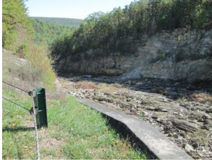
Figure 4.3.2.5.21: Long Pine Run Dam Spillway
