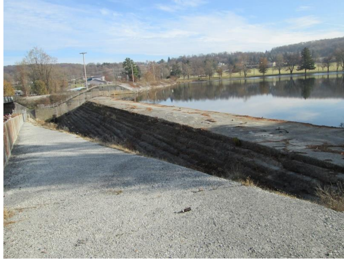
Figure 4.3.2.5.29: Lower Lake Royer Dam Spillway
