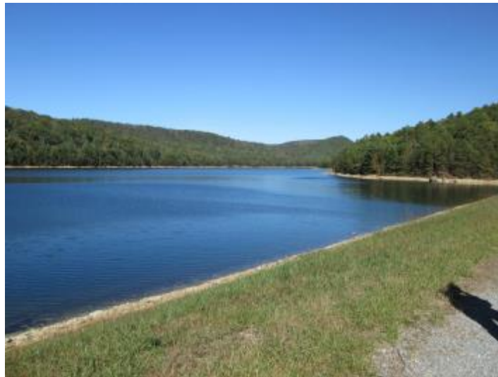
Figure 4.3.2.5.20: Long Pine Run Dam Entrapment Area
