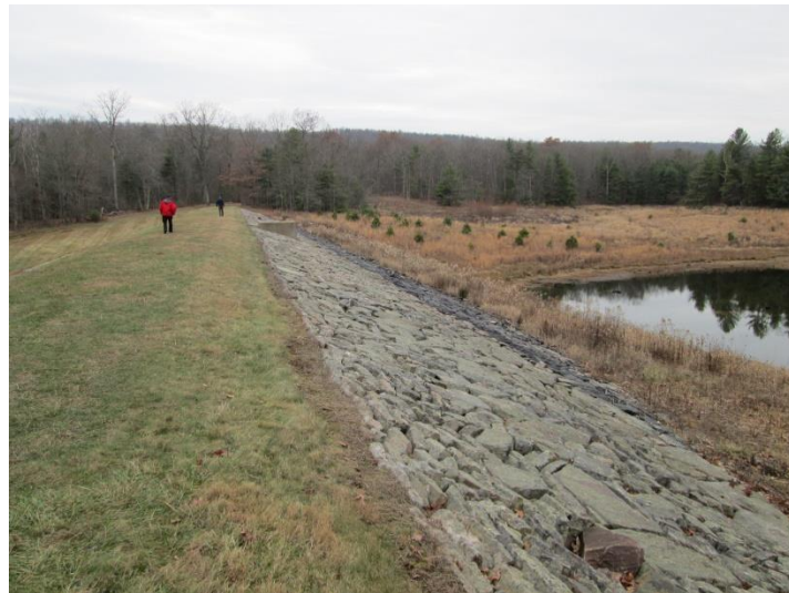
Figure 4.3.2.5.26: Meadow Grounds Dam Wall
