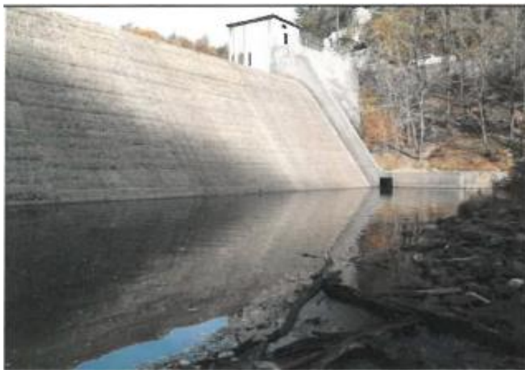
Figure 4.3.2.5.5: North Wing Wall of Roxbury Dam
