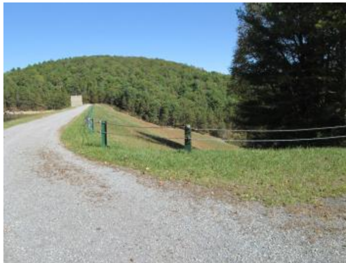
Figure 4.3.2.5.22: Long Pine Run Dam Wall
