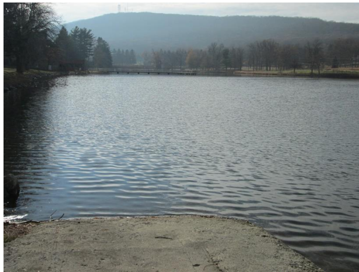
Figure 4.3.2.5.28: Lower Lake Royer Dam Entrapment Area
