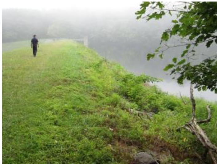
Figure 4.3.2.5.14: Antietam Dam Wall
