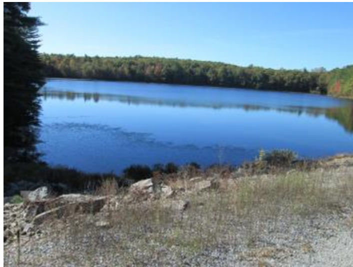
Figure 4.3.2.5.16: Carbaugh Run Dam Entrapment Area
