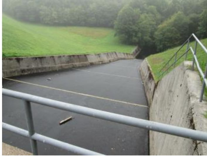
Figure 4.3.2.5.13: Antietam Dam Spillway
