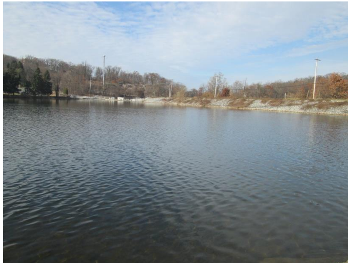
Figure 4.3.2.5.30: Lower Lake Royer Dam Wall
