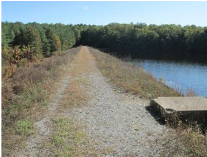
Figure 4.3.2.5.18: Carbaugh Run Dam Wall
