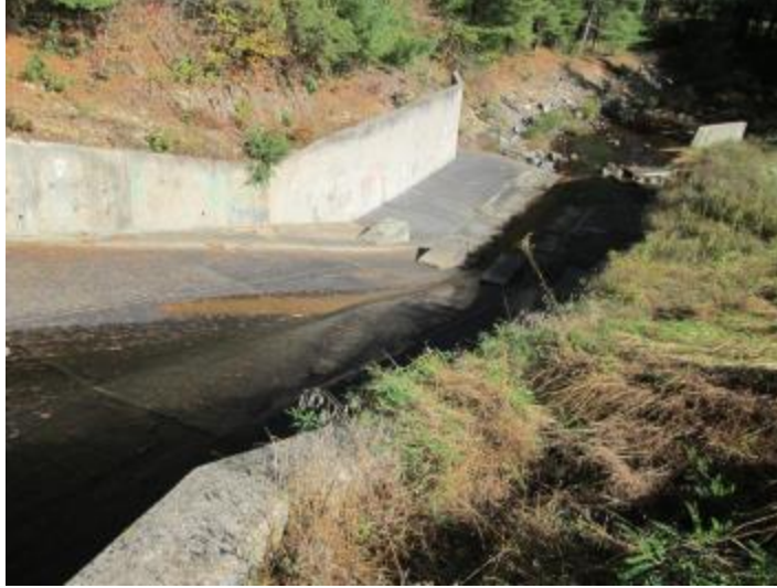
Figure 4.3.2.5.17: Carbaugh Run Dam Spillway
