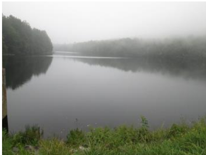
Figure 4.3.2.5.12: Antietam Dam Entrapment Area
