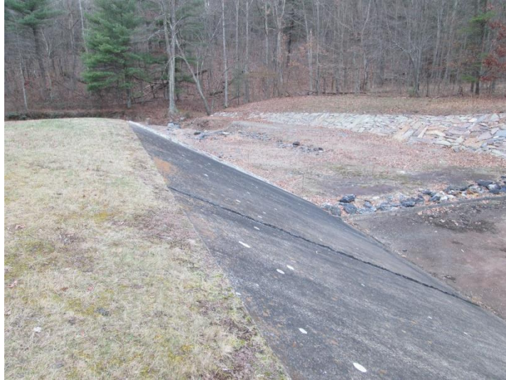
Figure 4.3.2.5.25: Meadow Grounds Dam Spillway
