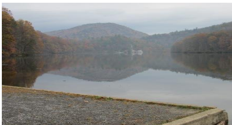
Figure 4.3.2.5.6: Entrapment Area of the Roxbury Dam
