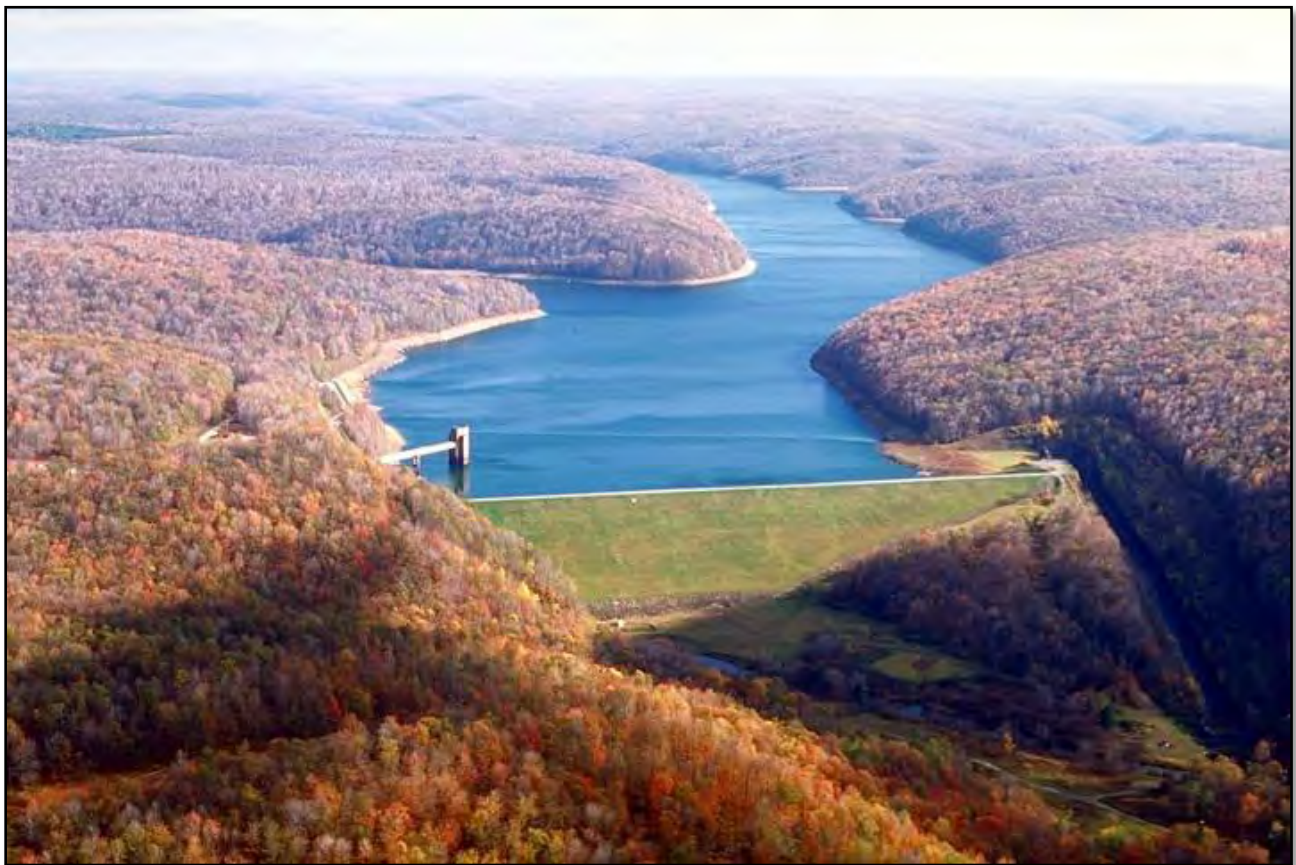
Figure 4-5: East Branch Dam. Courtesy of the US Army Corp of Engineers, Pittsburg District
