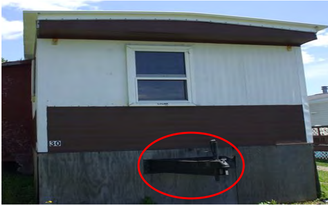
Figure 4-29: Mobile home or "trailer". Note the hitch attached to the front for towing.
