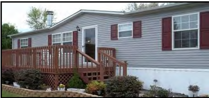
Figure 4-30: Manufactured home. No hitch attached but note the skirting around the bottom. This is typical in order to hide where the wheels are located.
