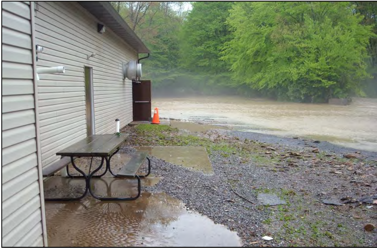
Figure 4-17: Jay Twp. VFD is surrounded by flood water. Pictured is the rear of the fire station. Luckily, the fire department's loss was limited to clean up costs only. The Jay Township Fire Department is located in Flood Zone A according to FEMA Flood Rate Map.
