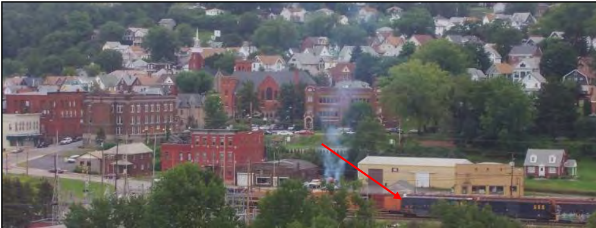
Figure 4-42: Train rail yard in Johnsonburg. Red arrow depicts location of the train in the foreground. Note the numerous residential properties in the background.
