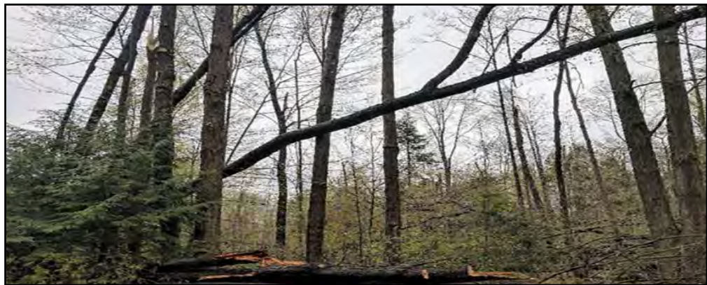
Figure 25: Tornado Clean-Up- The instability of this type of damage creates hazardous conditions for those tasked with the clean-up.
