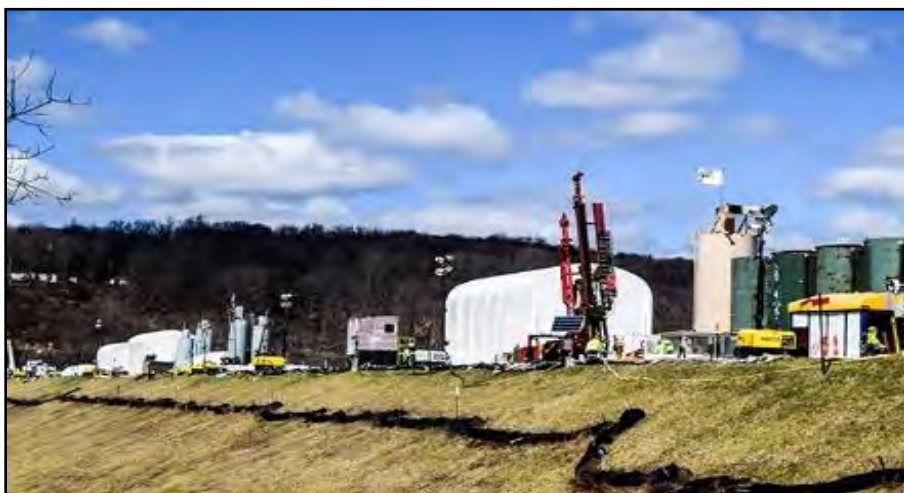
Figure 4-3: Work on the East Branch Dam Repair Project
