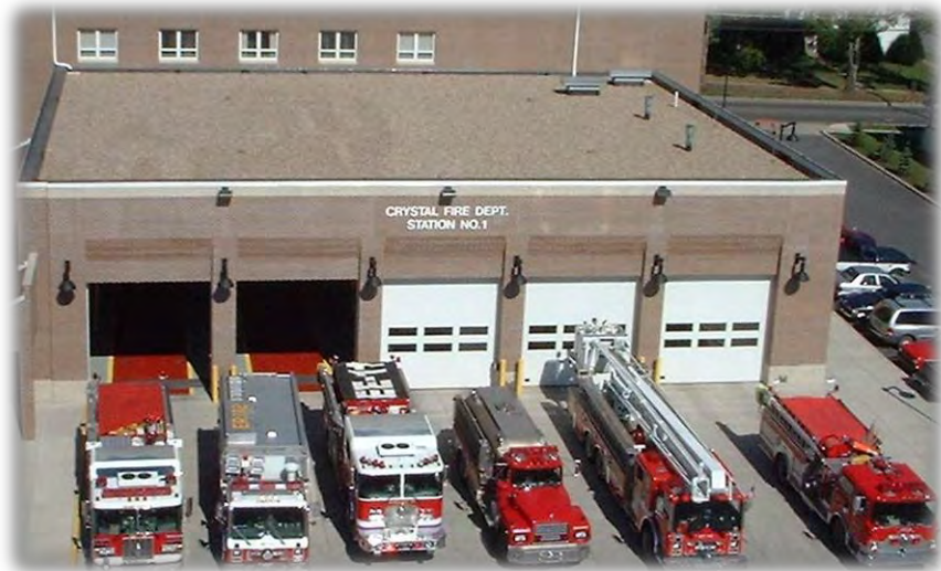
Figure 4-61: Crystal Fire Department, Station #1. St. Marys, PA
