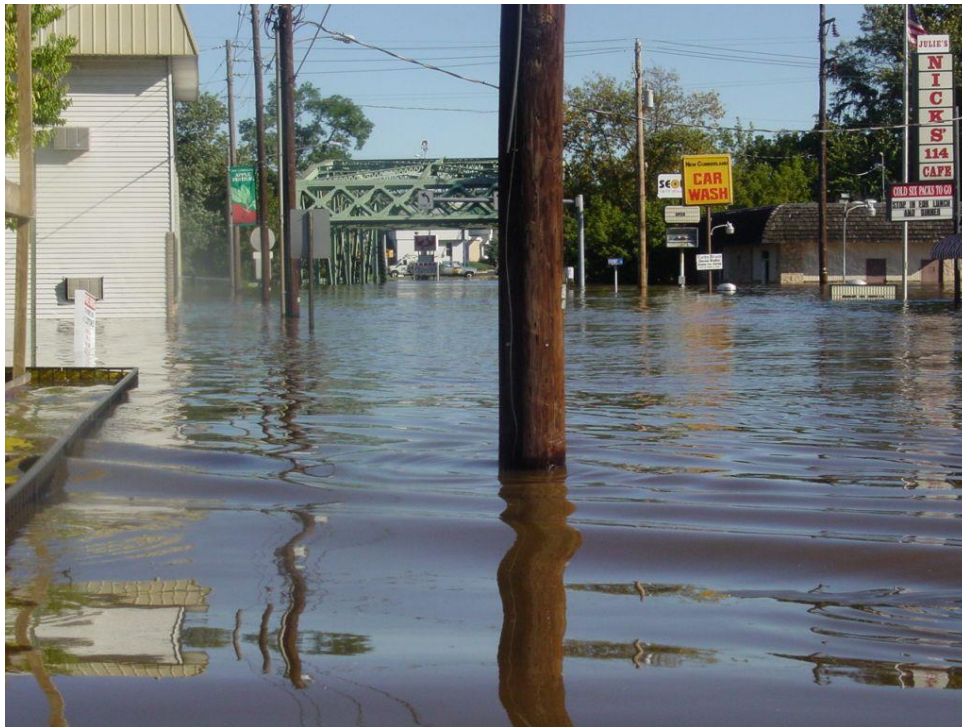
Figure 4.3.3-7: Flooding in New Cumberland, PA (Photograph courtesy of Cumberland County Department of Public Safety).
