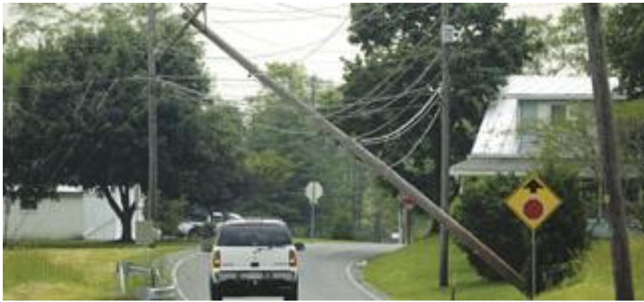
Figure 4.3.17-1: A telephone pole was leaning at the intersection of Bernheisel Bridge Road and Sherwood Drive in Middlesex Township, Cumberland County, PA on May 28, 2011 following a storm that caused power outages for thousands of county residents (Photograph courtesy of Jason Malmont/ The Sentinel , 2014).
