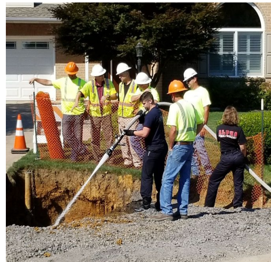
Figure 4.3.10-4: Workers repair sinkhole in Ferguson Township (Muthler & Hartley, 2018)
