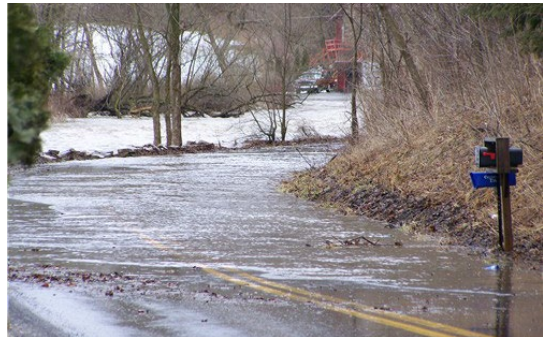
Figure 4.3.4-5: Flooding on Spring Creek Road in Bellefonte During Heavy Rain, March 5, 2008 (Accuweather, 2008a)
