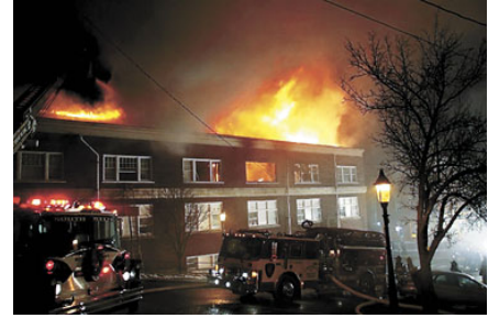
Figure 4.3.24-1: 2009 Fire at the Cadillac Building in Downtown Bellefonte (The Express, 2009)
