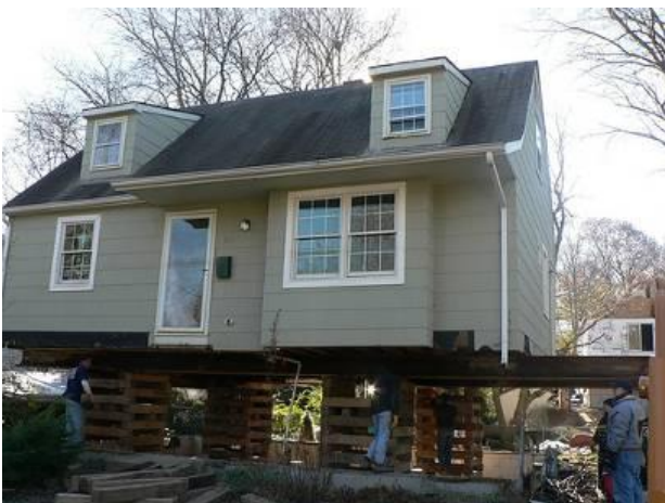
Figure 6.1-2 Yardley Borough Elevation Project
