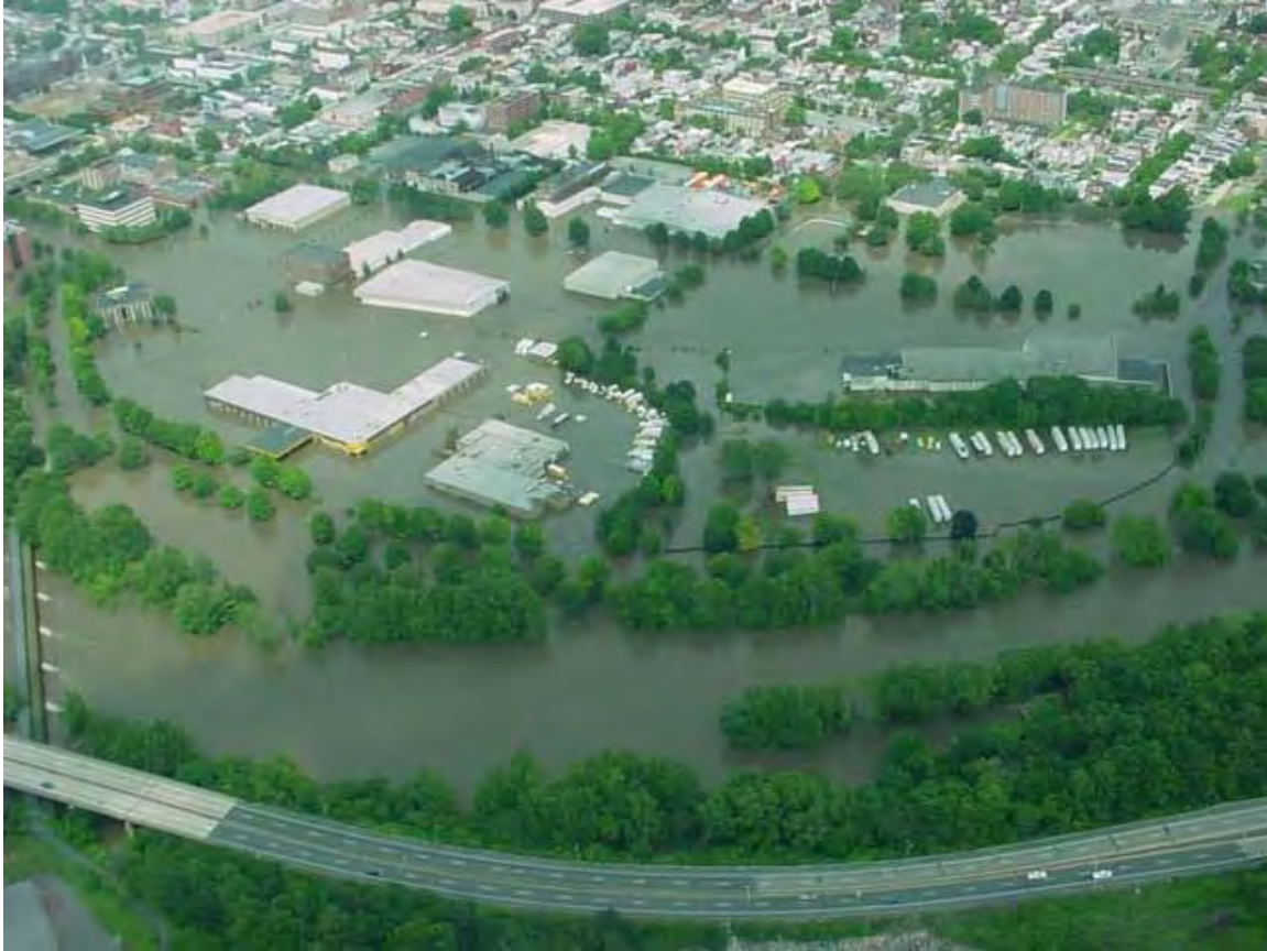
2006 Flooding in Reading City along the Schuylkill River
